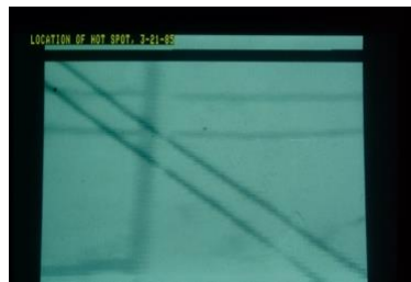
5-13. Single frame from thermal video images taken from helicopter of power lines.
